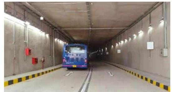
remote gates area of the expanding passenger terminal,” the statement added. “The GSE tunnel will minimize time loss during crisscross movement of airlines and GSE operations vehicles, equipment, passenger coaches required for turnaround of flights, resulting in fuel saving... The annual savings of the carbon emission with this newly built GSE tunnel would be about 7000 tons per annum,” GHIAL says.
